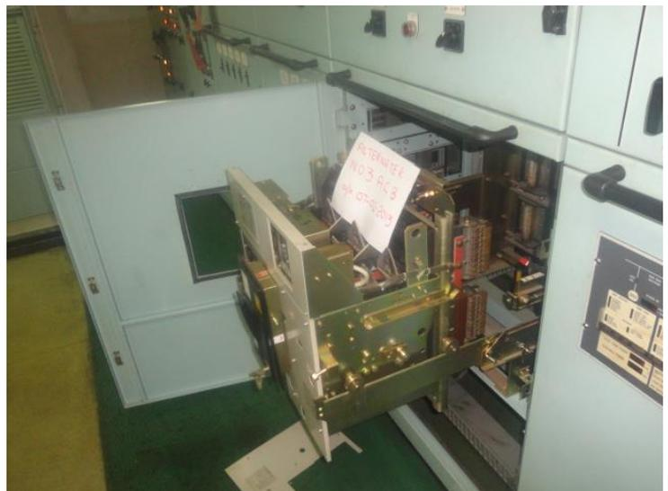
The main contact closing pressure is kept high so that the temperature rise in the contacts while carrying current remains within limit. Closing coil operating on D.C voltage from a rectifier is provided to close the circuit breaker by operating a push button.
